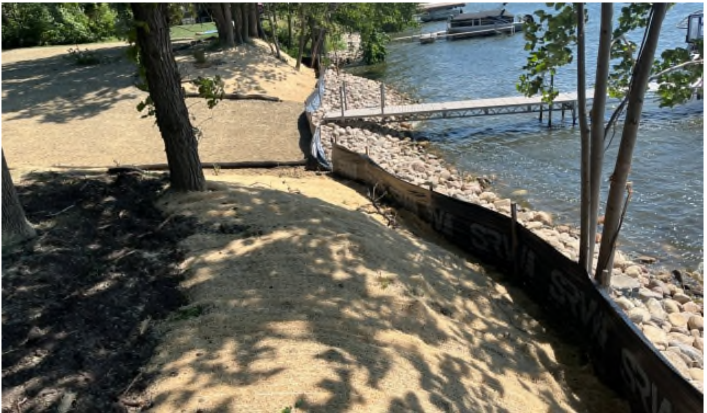
Erosion blanket installed, plugs and trees/shrubs planted
