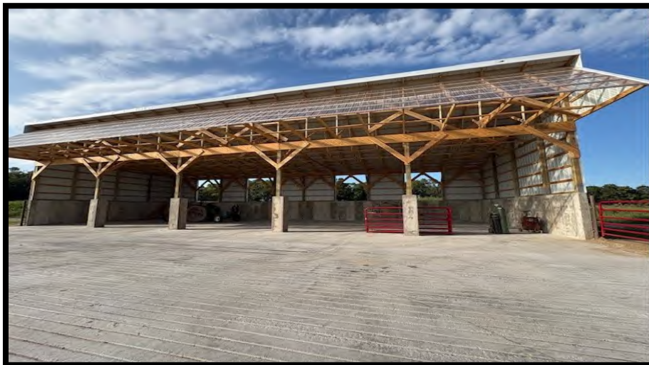
2026 Solid Manure Storage Stacking Slab
