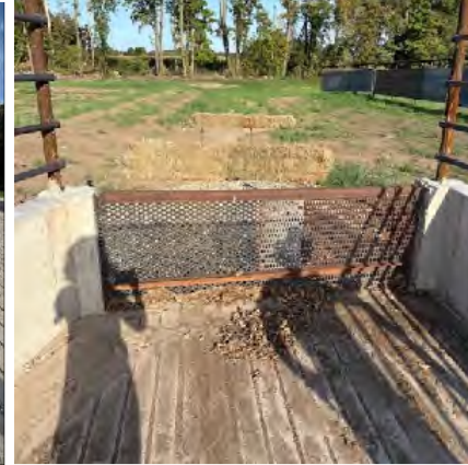
Hog panel that allows liquid to flow but traps solids.
