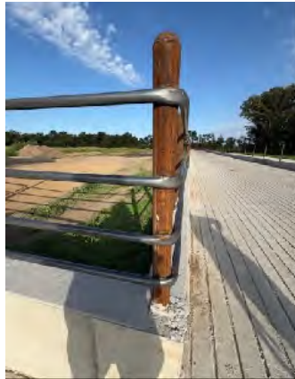
Heavy duty reinforcement along two foot wall.
