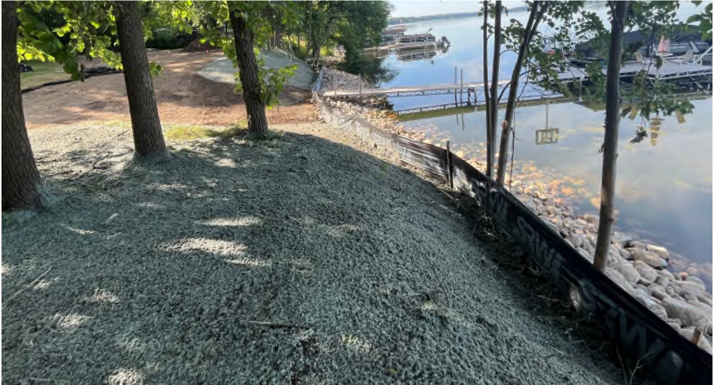
Rock installed and buffer seeded
